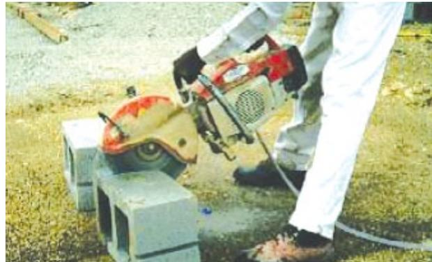
*A worker cutting concrete block using a handheld saw that applies water to the blade. The water reduces the amount of silica-containing dust that gets in the air.*
